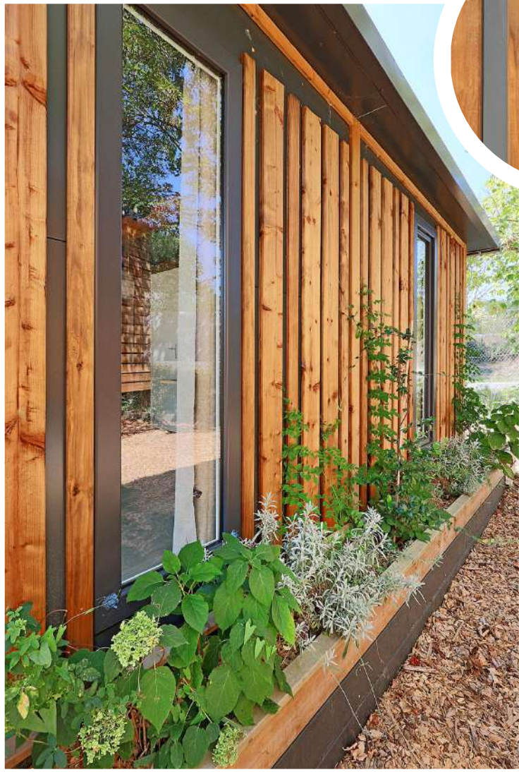
openwork wood cladding and plant integration
