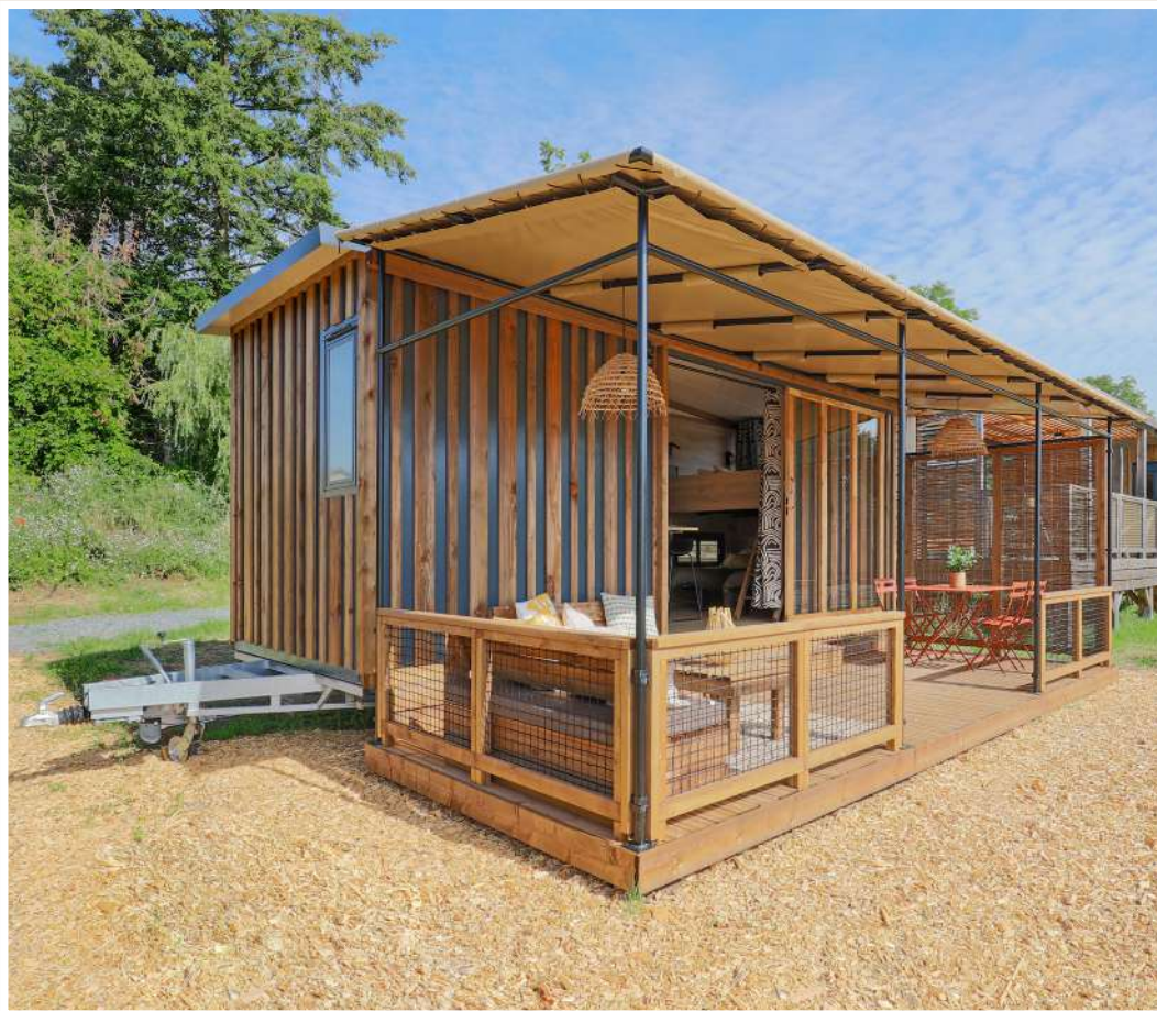
Constrained areas & mobility → chalet on wheeled chassis
